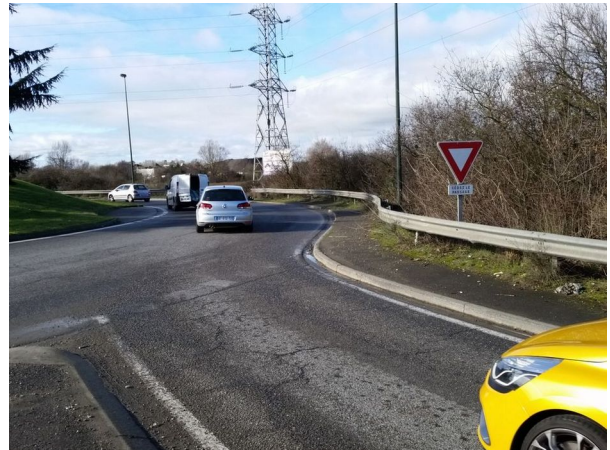
Figure 7: Le rond-point de raccordement à l'autoroute
